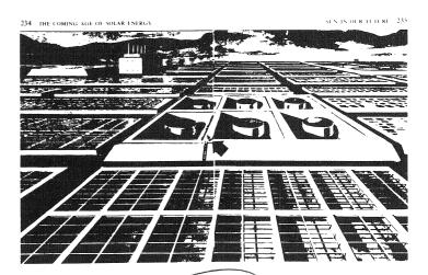
Artist's impression of a solar power plant. Arrow points to a human figure, dwarfed by its surroundings. A 1,000 MW fossil-tired or nuclear plant can be built on a few acres; a 1,000 MW solar plant would need 50 square miles of collecting area. No technological advance can ever change the dilute solar influx of 1 kW/m<sup>2</sup>.
